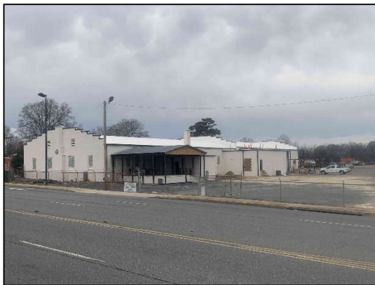
A commercial building undergoing rehabilitation bordering the site to the north
